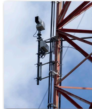
*The Firewatch camera system is mounted to a City of Austin communications tower on Mount Larsen, just north of West Lake Hills. Camera images are relayed to our dispatch center using wireless radio signals.*
